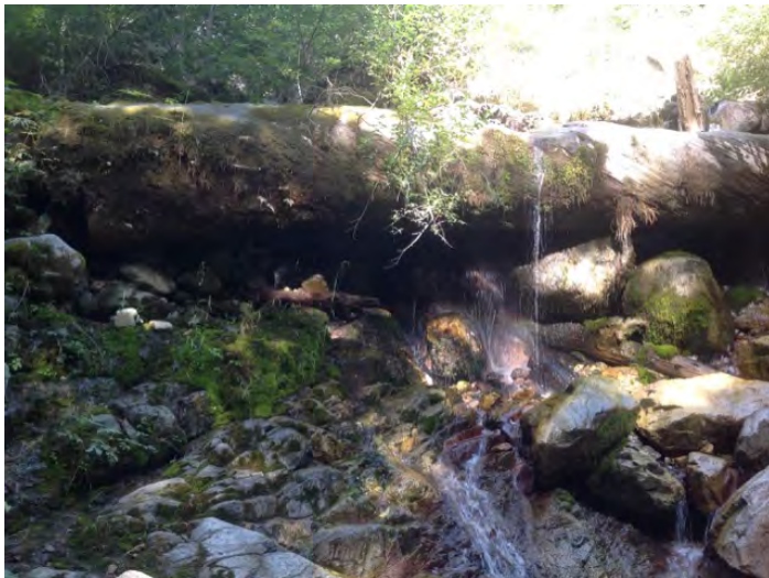
log retaining fill on fillslope
