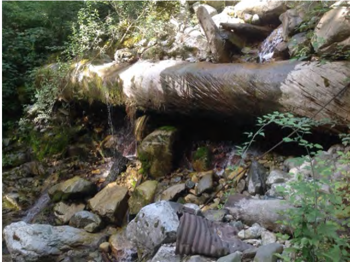
log retaining fill on fillslope
