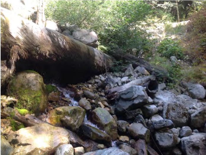
left bank of fill retaining log - tied into bank
